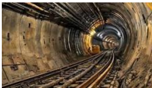
Figure 18. Utility Corridor along Subway Tunnels.
